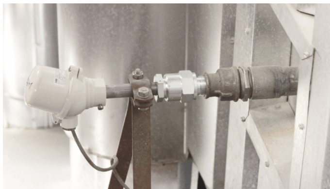
Figure 4: High temperature thermometer in the furnace
