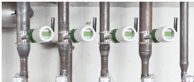
Figure 14: Temperature sensor for surface mounting, with integrated Energy Harvester
